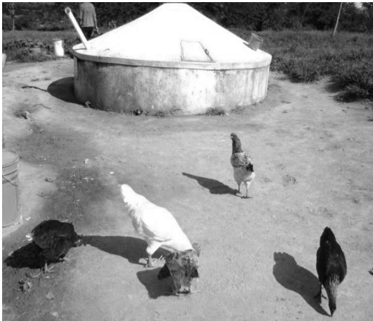
(a) Cisterna CE2.
